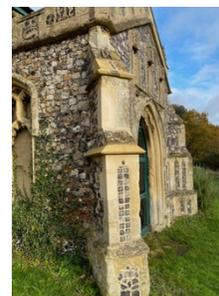
continue into 2024 and beyond. One of the buttresses at the front of the porch has been repaired by a master stone mason, as has the stone work to the lancet window on the south face of the tower and the louvres in the upper west window have been replaced. Inside the church the bell chamber and sounding chamber have been repointed and part of a wall in the history room has been replastered. The cost of the work to date
